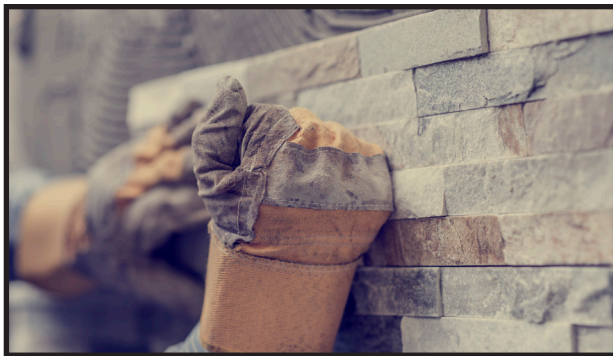
Tenon® Masonry Veneer Mortar PM can be used for both traditional thick bed scratch and base coats and as bonding mortar
